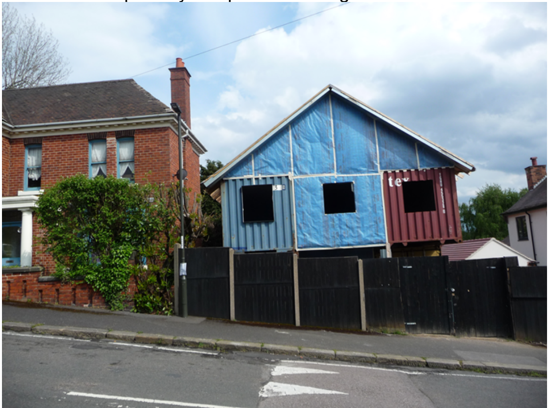
Photo to show partially completed dwelling
